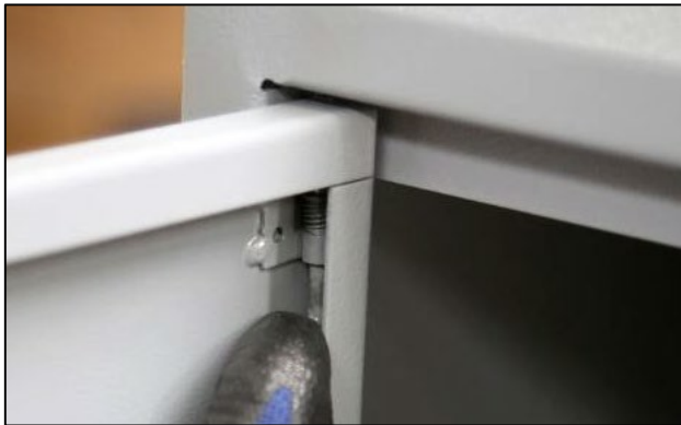
Illustration: Removing the switch box door
